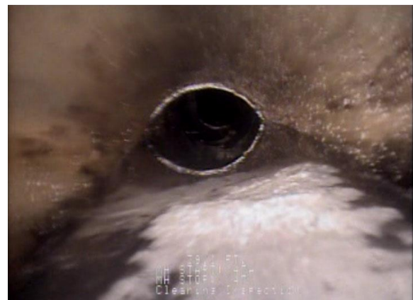
Severe sag in VCP main. The camera was unable to continue through this sag
